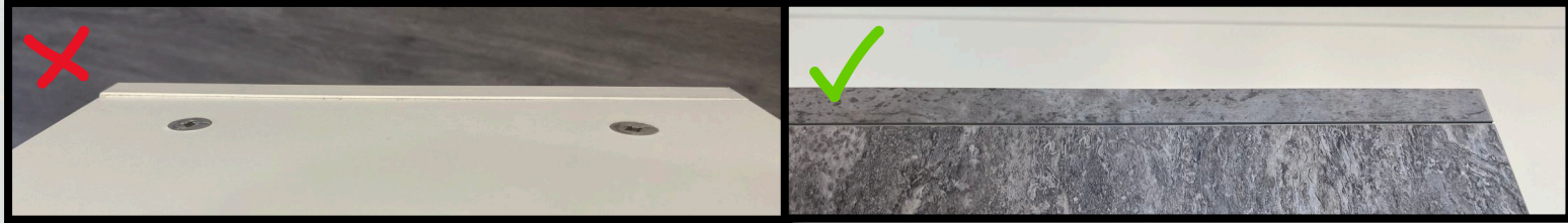
4.) alignment at the joints of carcass boxes,
